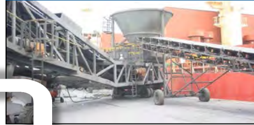
Hopper to Stockpile
